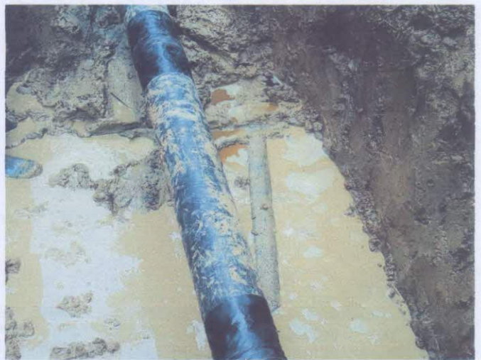
FIG F: Incident point after repairs
